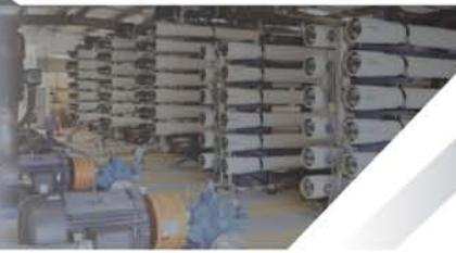
by digging independent brackish wells to feed these RO units at Water Filling stations at Jabriya and Omariya and plans to continue to install RO units for all the water filling stations sites.
